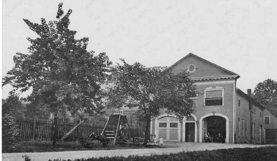
Old Edgewood Municipal Building
